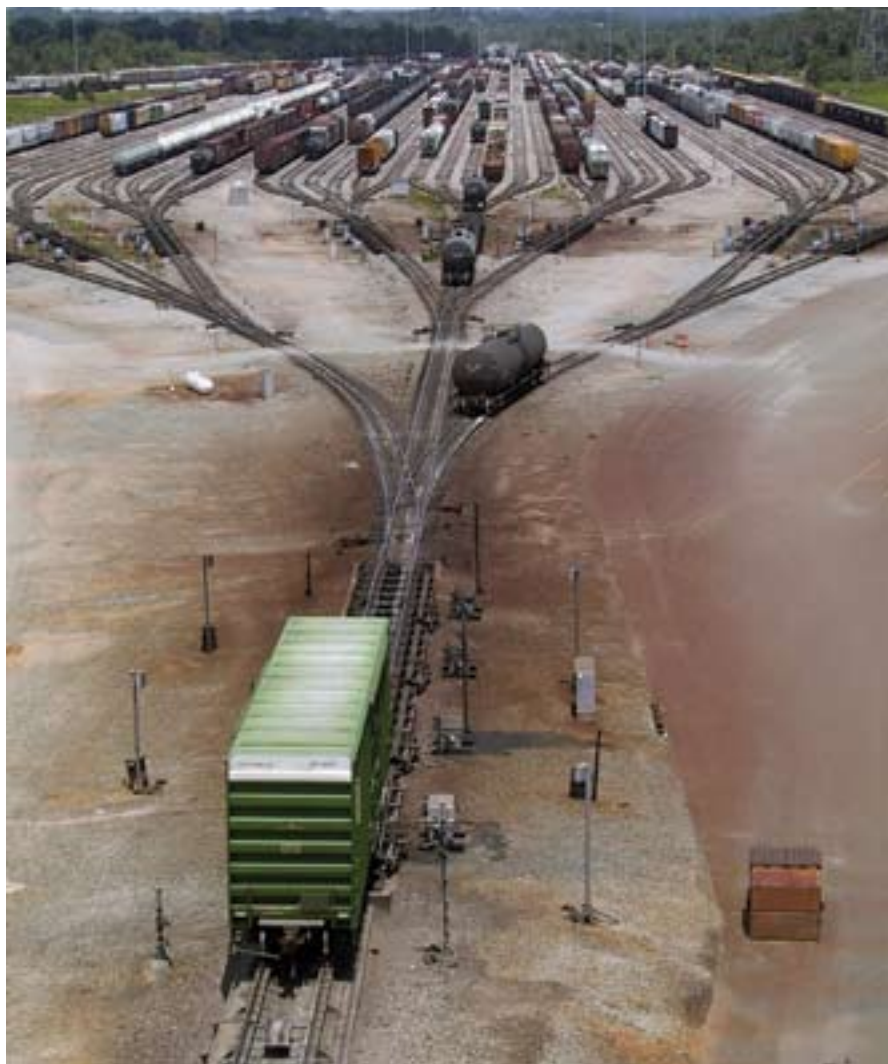
Rail cars roll off the hump and into the classification tracks of a freight yard in Linwood, North Carolina, operated by the Norfolk Southern railway. The yard sorts cars onto more than 40 tracks in order to assemble trains bound for various destinations. As each car rolls down a slight grade, a computer identifies it from a radio-frequency tag, regulates its speed and sets the switch points according to the car's destination. (Photograph by the author.)
