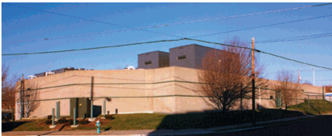
Figure 3. A windowless concrete building in southern New Jersey may or may not be a Network Access Point.
