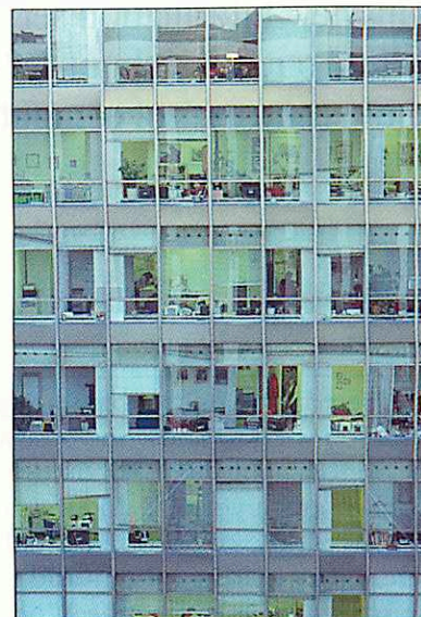
Glass-wall architecture reveals the underlying office building grid.
