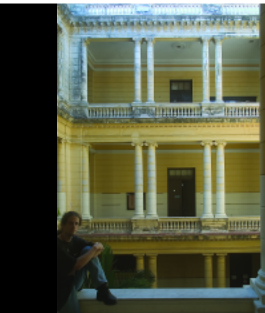
At the faculty of physics, the columns are stately, but chunks of masonry are falling into the courtyard below. At left is Roberto Mulet, a former student of Altshuler, now assistant professor.
