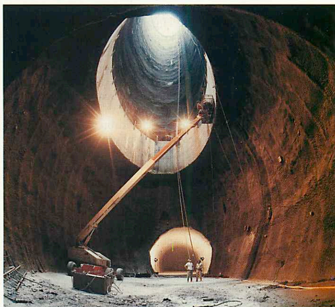
Excavation of the 54-mile tunnel begins at the Texas site of the Superconducting Super Collider.
